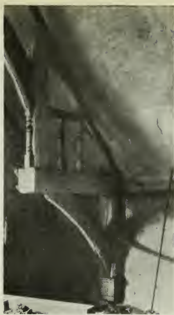
SAFFRON WALDEN. (4). Abbey Farm, Roof Truss in Chapel ; c. 1600.
